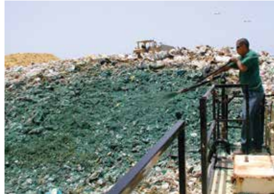
Dyed green to confirm coverage rate for efficiency, unlike non-dyed spray-on products
