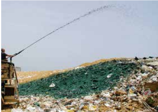
Upon application forms a consistent and effective layer between waste and the surrounding environment
